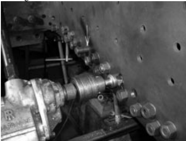
Countersink tool at work
