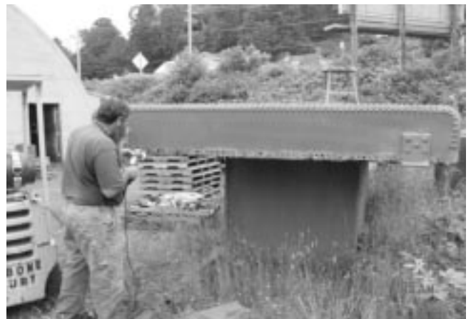
Casey removing corroded rivets
