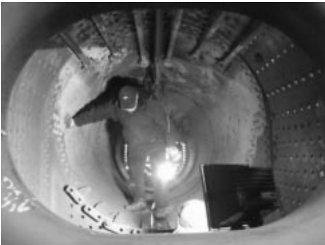
Inspecting the boiler
